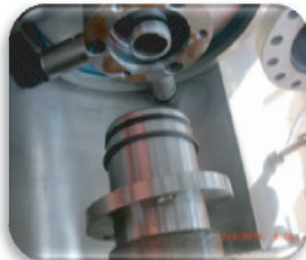
The required number of UNIT 2 elements are sequentially installed.
